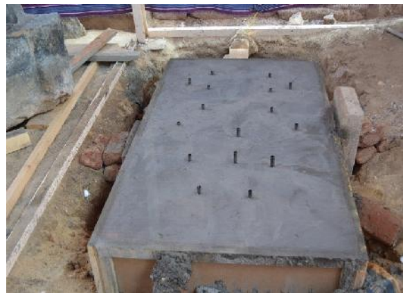
Figure 10: Excavation for the Sekhmet Statue base Figure 11: The Completed Concrete base.
