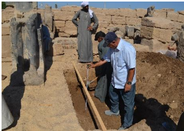
Figure 10: Excavation for the Sekhmet Statue base Figure 11: The Completed Concrete base.
